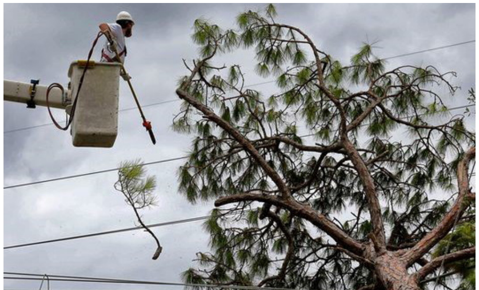
Lineman conducts vegetation management of power lines.
